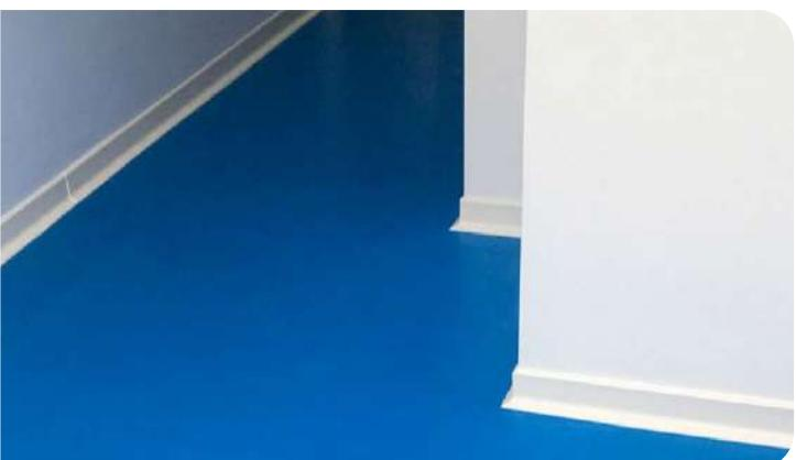
PolySto prefabricated **PV15F** full core PVC skirting installed against a FRP embossed sheet, finished with HygiSeal.
