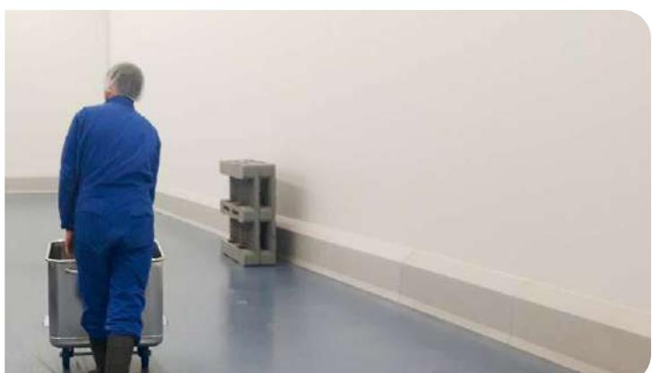
PolySto prefabricated **IP40F Natural** CleanRock kerb.
