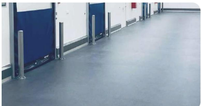
PolySto prefabricated ICS30F (left) and OCS30F (right) stainless steel kerb with concrete core installed on top of a concrete or cast floor.
